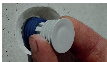
Position the Sealing Plug in the formwork spacer
